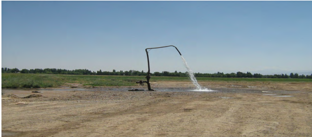
Photo 1: Groundwater source for construction dust suppression, Kulan By-Pass, June 2012
