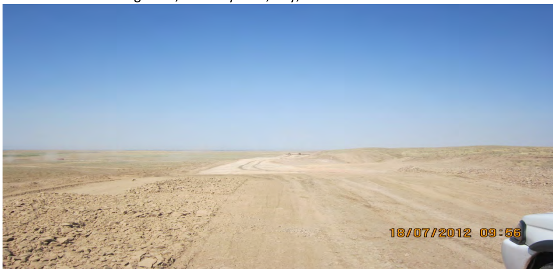
Photo 3: Earth work, Korday By-Pass, July 2012
