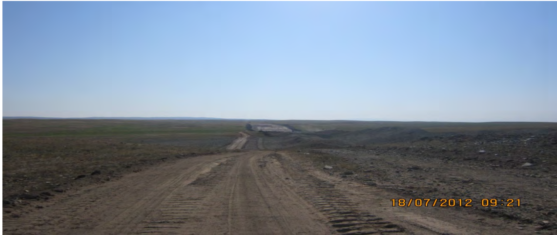
Photo 6: Stripping top soils, Korday By-Pass, July, 2012
