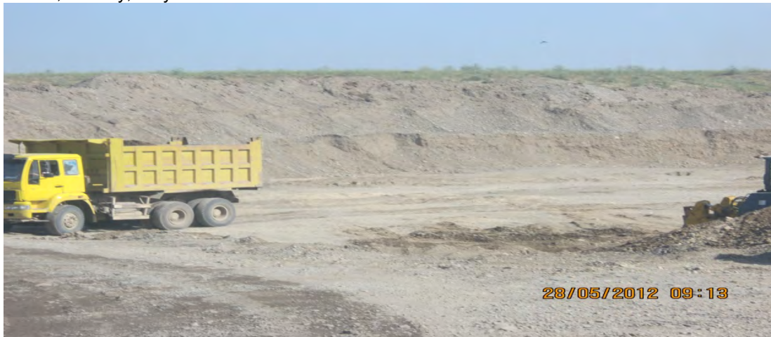
Photo 8: Excavation of Suitable Soil from Borrow Pit, Access to Kyrgys Border, Karday, May 2012
