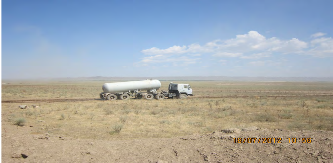
Photo 4: Water spraying for dust suppression, Korday-Bypass, July 2012
